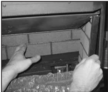
Figure 8.6 Install the left and right brick panels. Use the screw placement shown in Figure 8.3 to secure them in place. Reassemble appliance.
